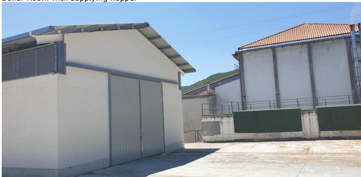
General view. In the foreground, chips storage plant. On the right, acces to the fidding chute together with the boiler room.
